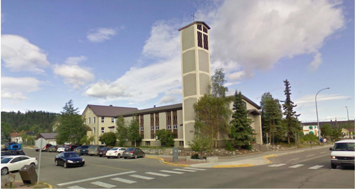
Figure 1: Sacred Heart Cathedral viewed from the southeast
